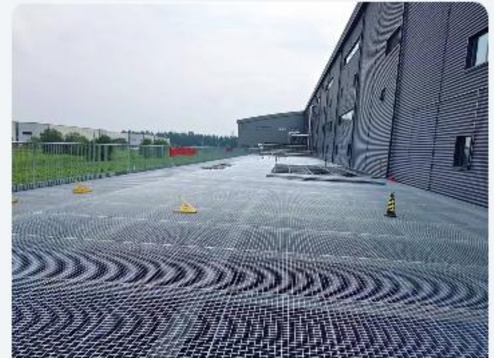
DATA & INDUSTRIAL FACILITIES
